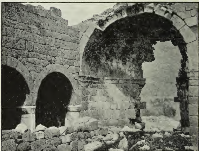
FIG. 19.—No. 4, interior of apse.
